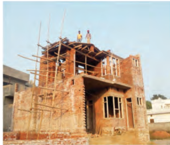
Masons making the building
