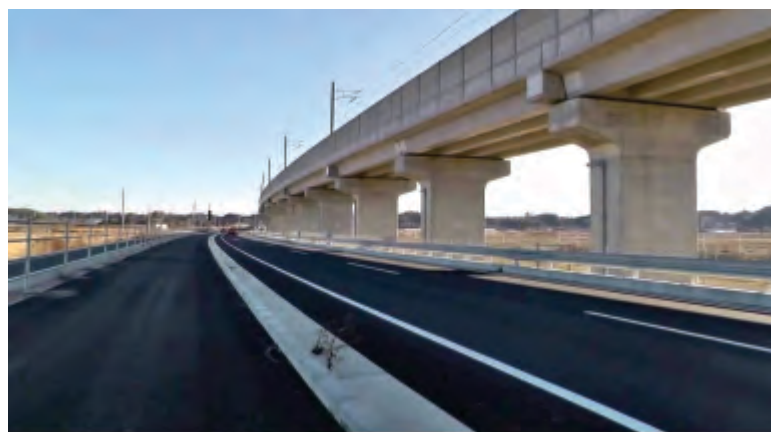
Fly over bridge
