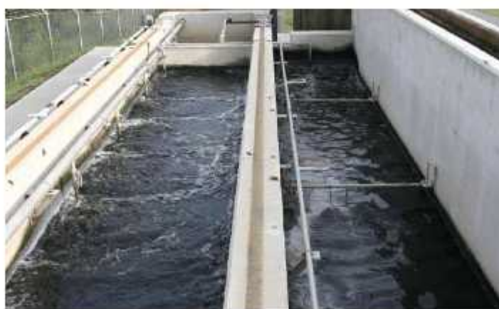
Fig 18.4: Grit and sand removal tank
