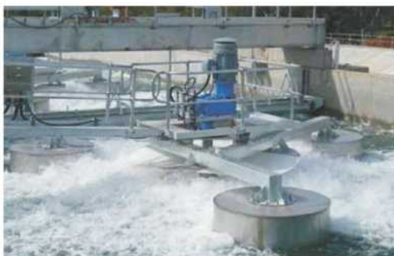
Fig 18.6 Aeration of clarified water
